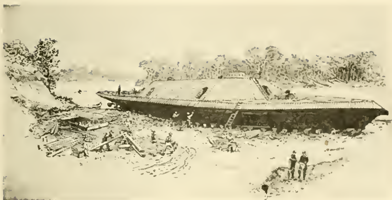
CONSTRUCTION OF THE ALBEMARLE
